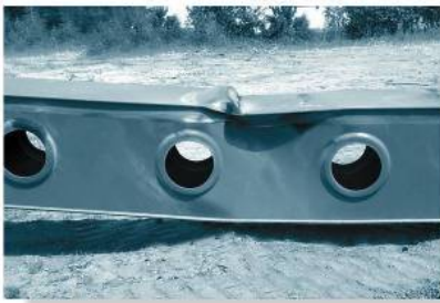
This crane boom failed by buckling caused by an overload. Note the region of localized collapse.
