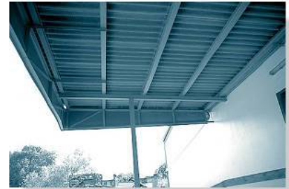
The design of a roof system requires a careful consideration of deflection. For example, rain can accumulate on areas of the roof, which then causes ponding, leading to further deflection, then further ponding, and finally possible failure of the roof.
