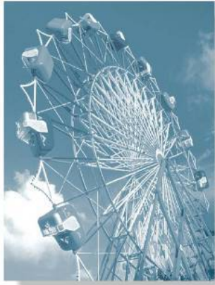
The design of members used for amusement park rides requires careful consideration of cyclic loadings that can cause fatigue.
