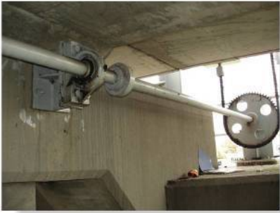
Long shafts subjected to torsion can, in some cases, have a noticeable elastic twist.
