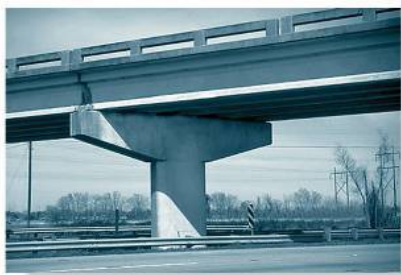
The beam for this bridge pier has a variable moment of inertia. This design will reduce material weight and save cost.
