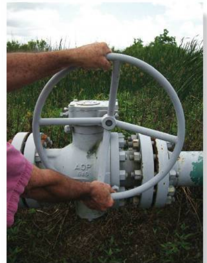
The shaft attached to the center of this wheel is subjected to a torque, and the maximum stress it creates must be resisted by the shaft to prevent failure.
